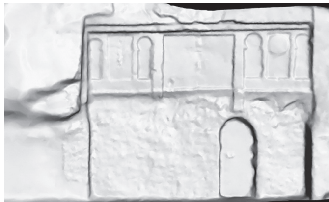
Fig. 7-8 Church of St John in Gülsehir: photo and mesh of the reconstructed image. The texture was removed to better understand the geometrical structure of the object. (B. Polimeni)
