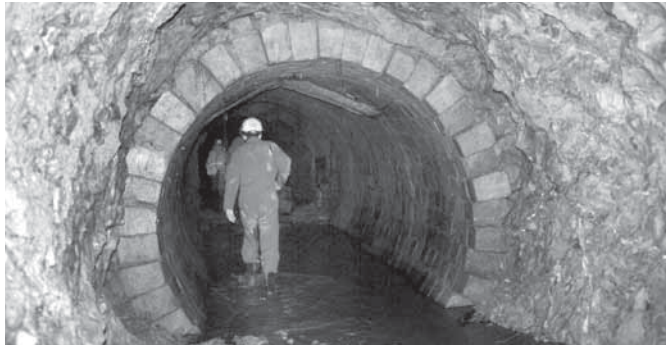
Fig. 4 Cinnabar mines in the Siele valley, Tuscany. Note the lithologic transition between lithoid rocks (marly limestone with good self supporting characteristics) and highly loading clay schist that needs walls coating (photo: S. Del Prete).
