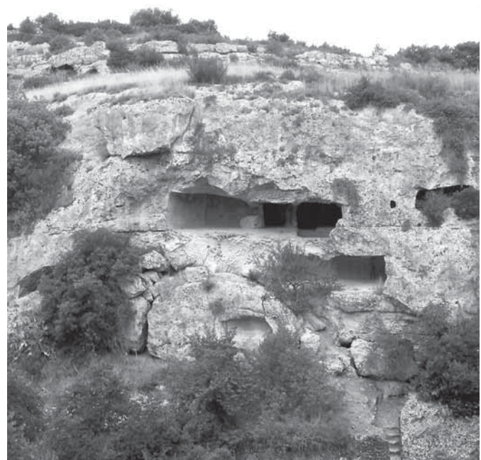
Fig. 16 Madonna della Scala (Massafra, Taranto): the rock failures on the right cliff of the ravine has damaged the caves (photo: M. Parise).
