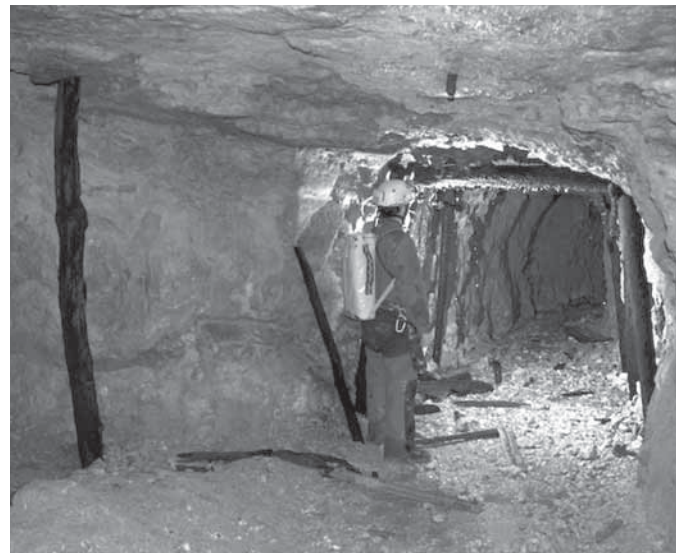
Fig. 5 The supporting structure for the vault in a bauxite mine (Cusano Mutri, Monti del Matese - Campania) is realized in correspondence with a karstic fracture (photo: N. Russo). The drip of the drainage through the same fracture is evident.
