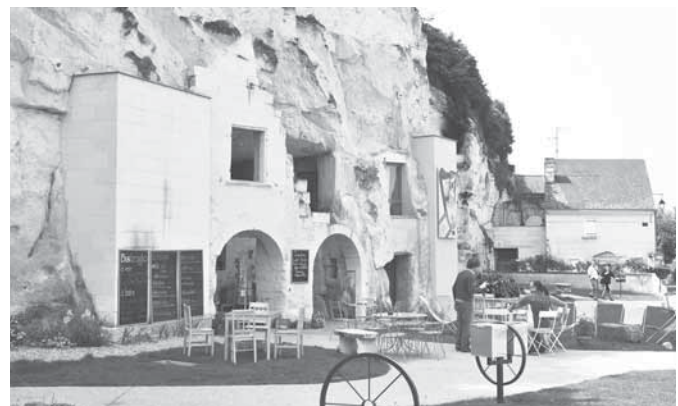
Fig. 9 Turquant hillside le bistrotroglo from the level of street Château Gaillard.
