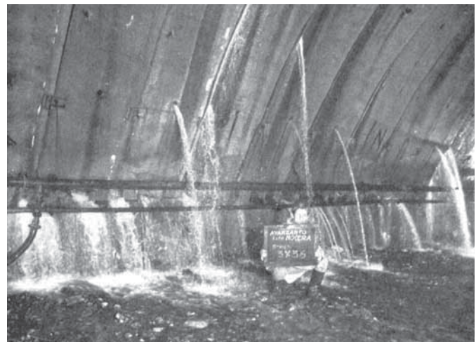
Fig. 6 Floods during the works for a railway tunnel, Nocera - Salerno (from Celico et al., 1977).
