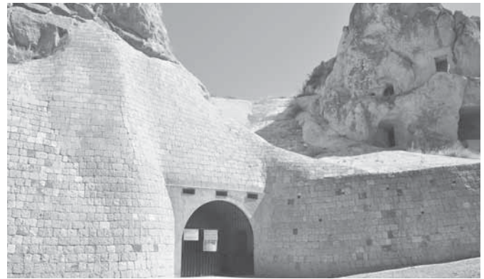
Fig. 29-30 Toakali Kilise and the Church of S. Barbara in Goreme. Examples of wrong conservation interventions.
