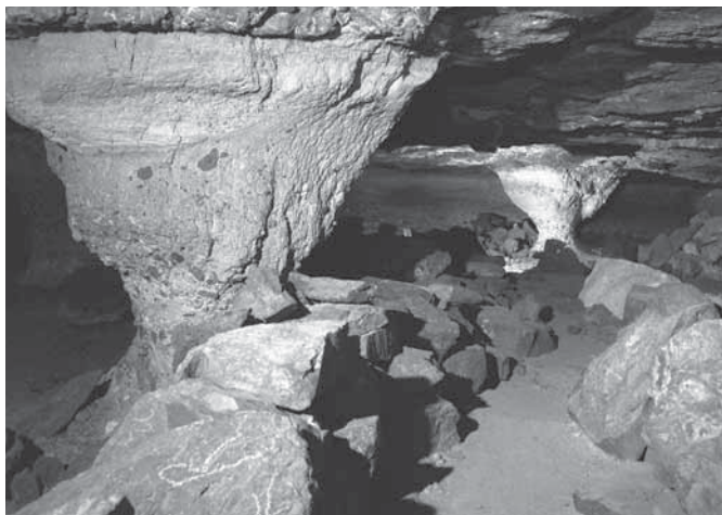
Fig. 15 Ani, Eastern Turkey. Thinning of pillars in an obsidian mine (photo: R. Bixio - Centro Studi Sotterranei). The typical splintering along the pillars is due to the vertical loads.
