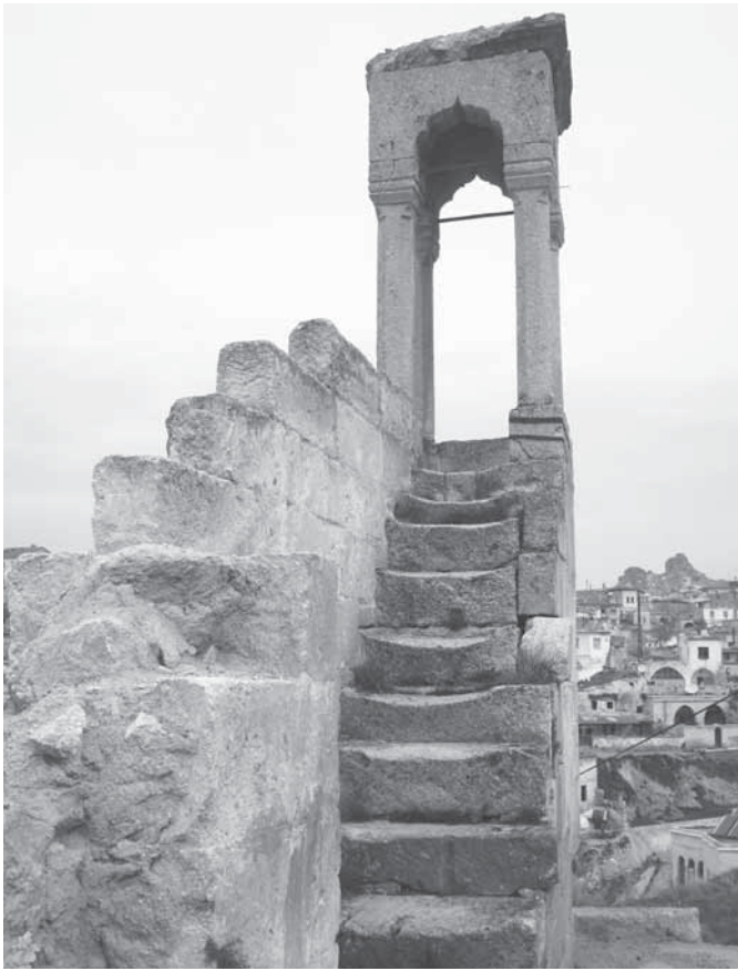
Fig. 15 Çukur Mosque, kiosk type minaret.
