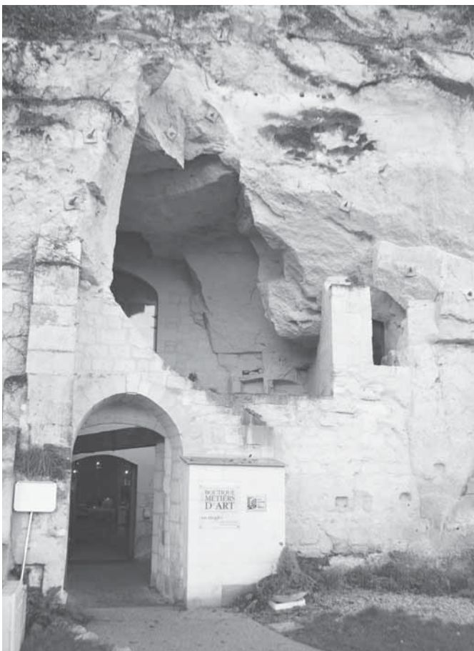
Fig. 13 Façade of the art craft workshop.
