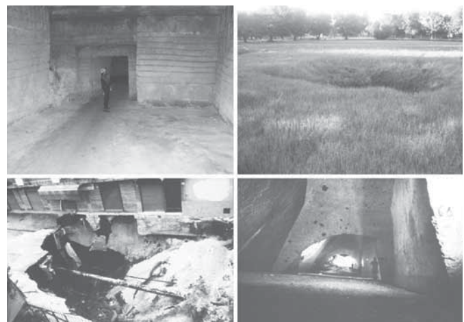
Fig. 18 Examples of underground cavities which have generated sinkhole phenomena (Cutrofiano, top, and Lusignano, bottom) causing, sometimes, serious damage to the overlying rural and urban settings (Cutrofiano photos: M. Parise; Lusignano photos: B. Bocchino, S. Del Prete).
