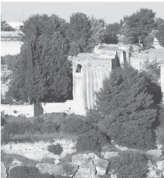
Fig. 4 The rupestrian church of Saint Andrea in the isolated tuff mass surviving to the extraction.
