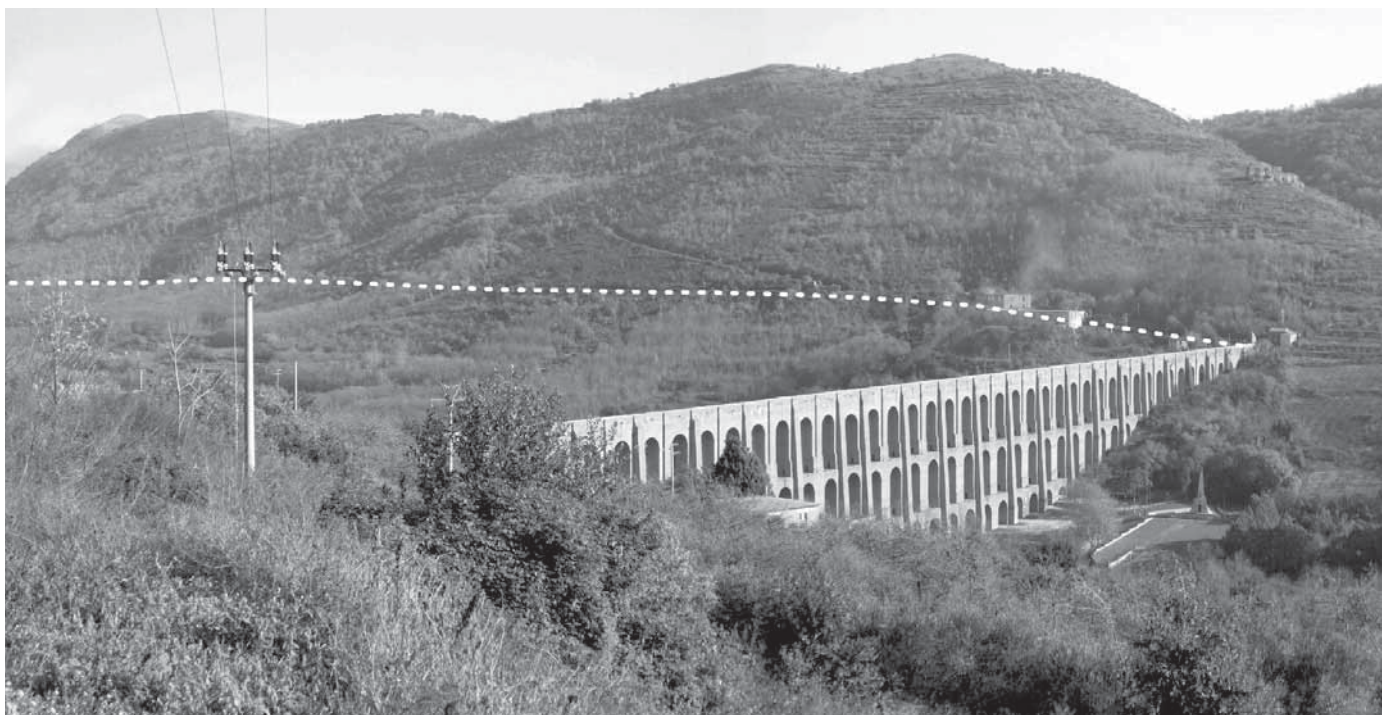
Fig. 1 Panoramic picture of the arched structure across Ponti della Valle valley; the broken line marks the hypogean track of the Caroline aqueduct along the flank of Longano hill, Caserta, Italy (photo: S. Del Prete).
