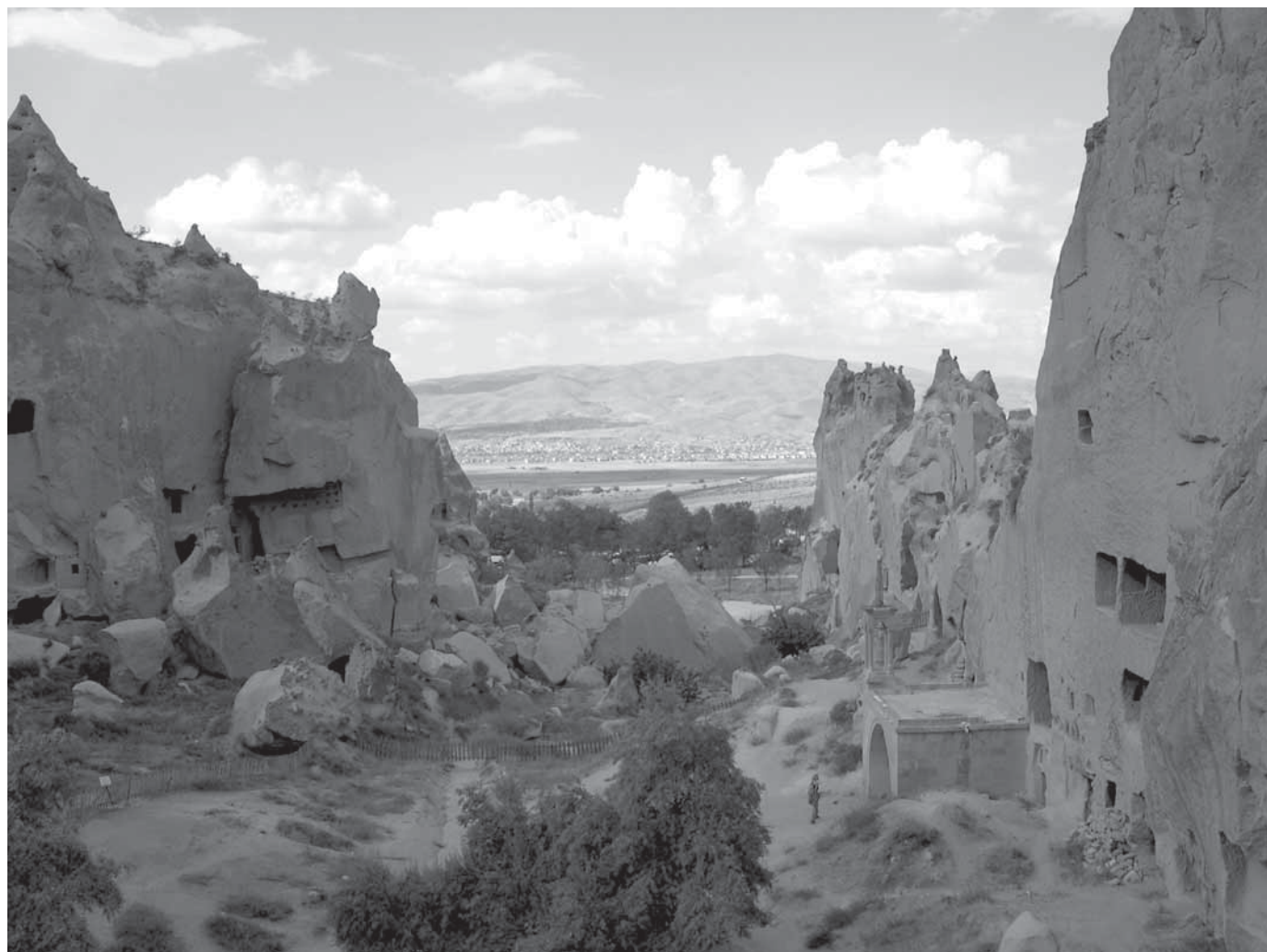
Fig. 19 Zelve. The wide de-tensioning fracture on the tuff cliff has revealed the underground rooms (photo: R. Bixio, Centro Studi Sotterranei). The evolution of the fracture will cause the collapse of this side of the cliff.
