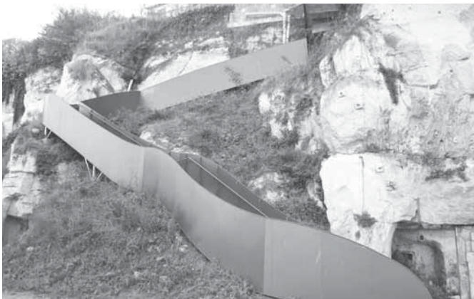
Fig. 12 Outdoor staircase of the hillside.
