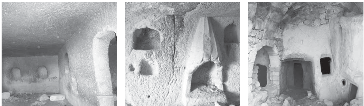
Fig. 5 Interior views of rupestrian houses.
